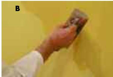
**2. Intermediate filling:** After the base filling is dried, approximately 300 g/m<sup>2</sup> of KEIM Stucco-Classico are applied in a "crosscoating" manner with a Stucco-trowel. Applying the filler manually mainly determines the final appearance of the surface.
