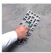
Prepare the surface with a grid-float before application of top coat render.
